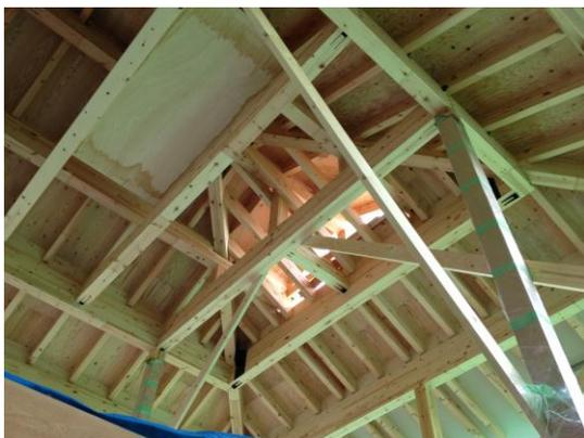
Fig. 18. Rear side of hipped roof
